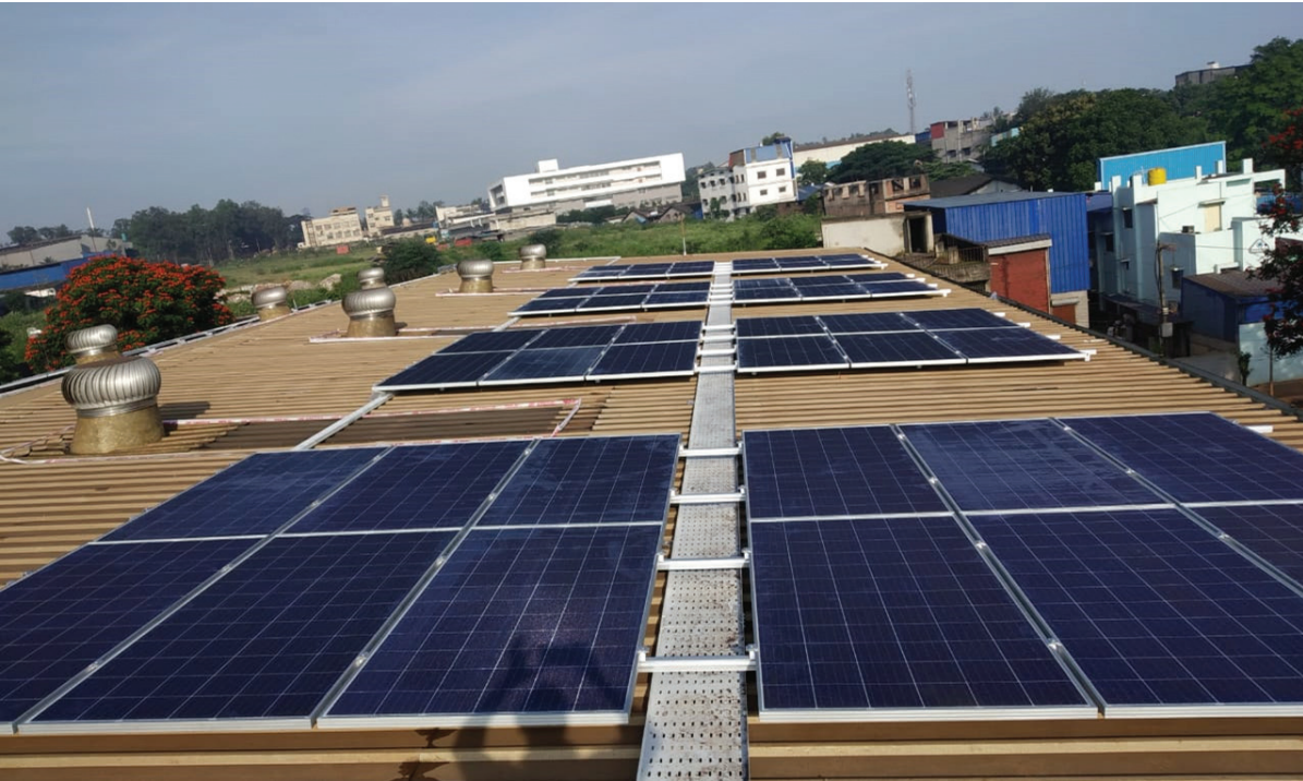
Figure 48: Rooftop solar PV system
