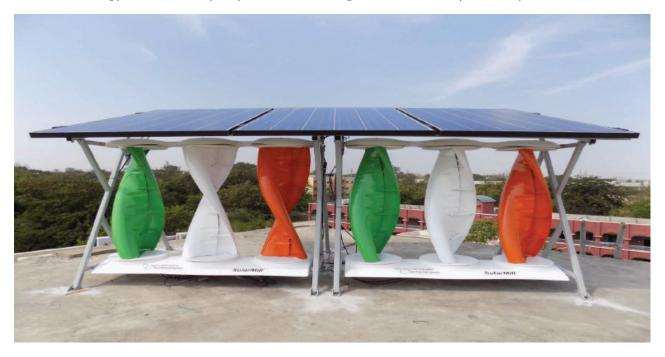
Figure 83: Solar-wind hybrid system
