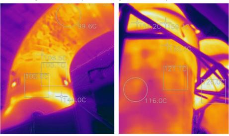
Figure 63: Thermal images of Hot gas generator duct connecting to cyclone separator
