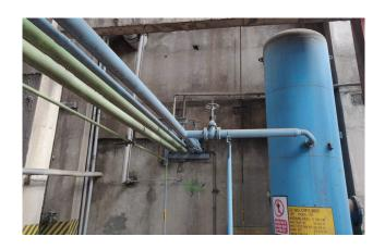
Figure 41: Existing compressed air piping
